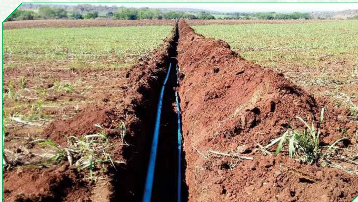
Picture 8: Installation of Correct Size Sub Mains at Mciniseli Tsabedze Farm
