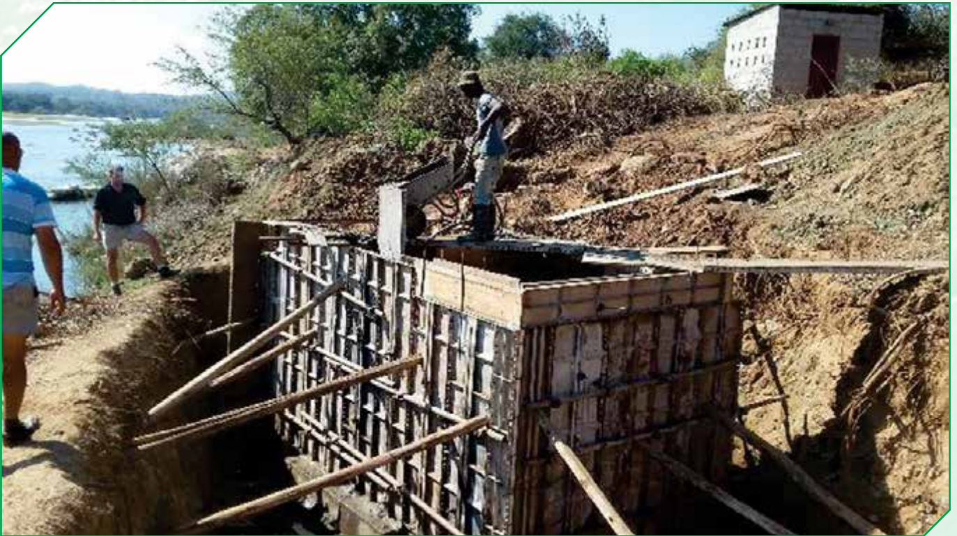
Picture 6: Construction of a Suction Sump at Mpilimbe Farmers Association
