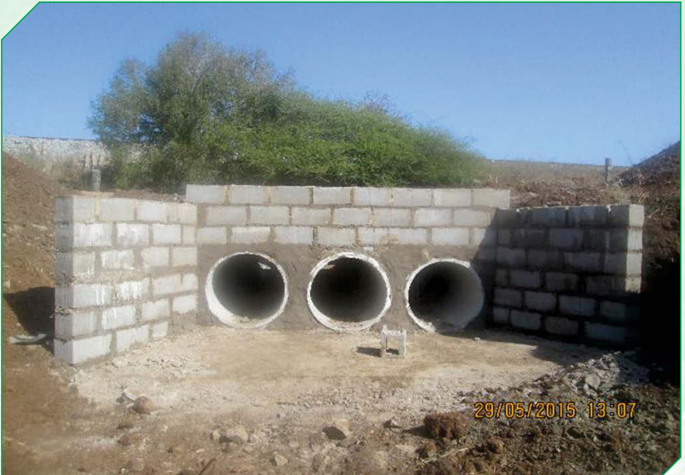
Picture 2: Culvert Construction at Makhulusihlengi farmers Association
