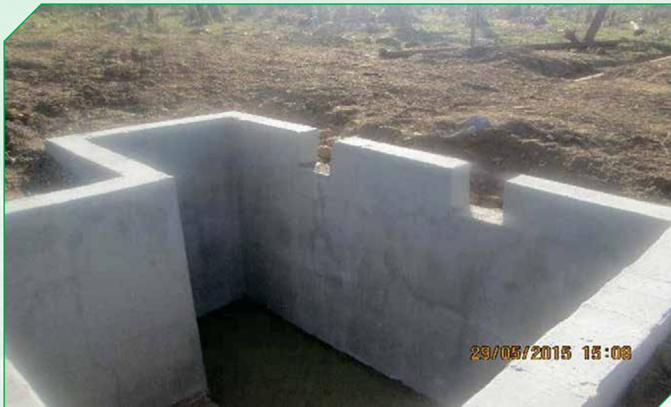
Picture 7: Suction pump at Construction at Nkambule Sugarcane Farm
